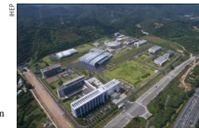
An aerial view of the CSNS facility in August this year.
